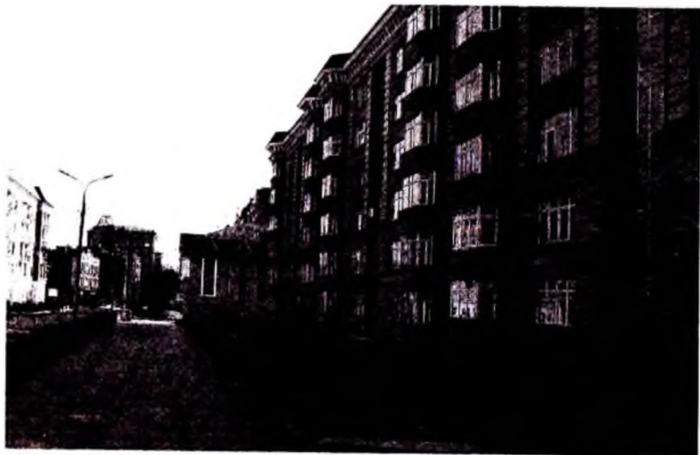
6.6-rasm. Toshkent shahridagi 6 qavatli zamonaviy turar-joy binosi
