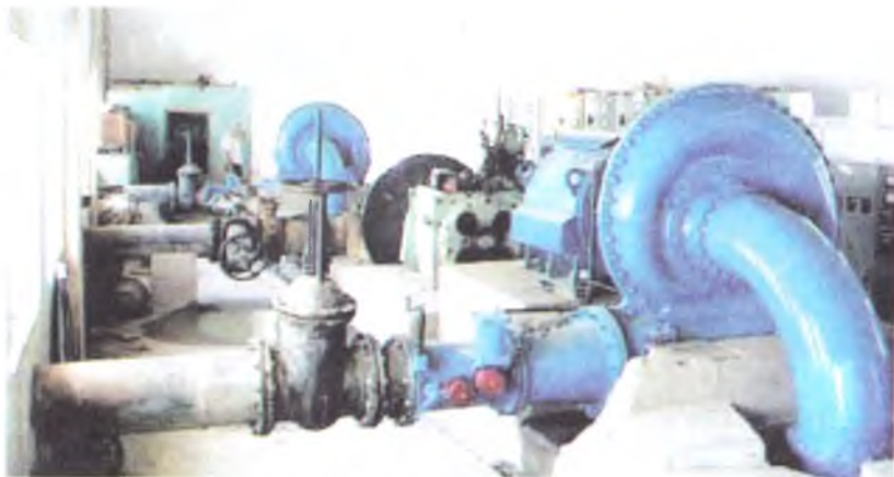
42-rasm. Gorizontial radial-o'qiy turbinalar o'rnatilgan kichik GES binosining ko'rinishi.
